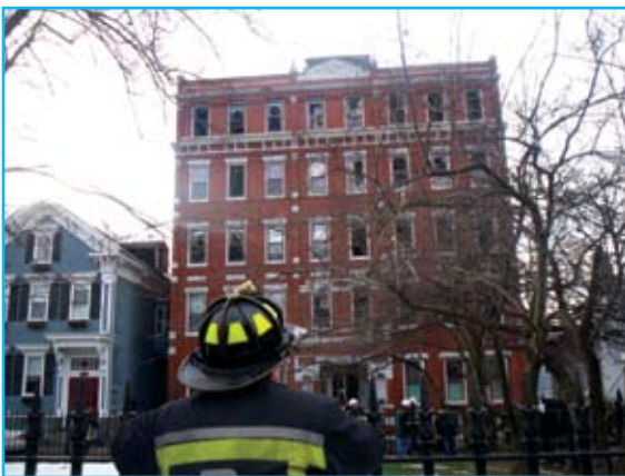
A view of the burnt building from the sidewalk.
